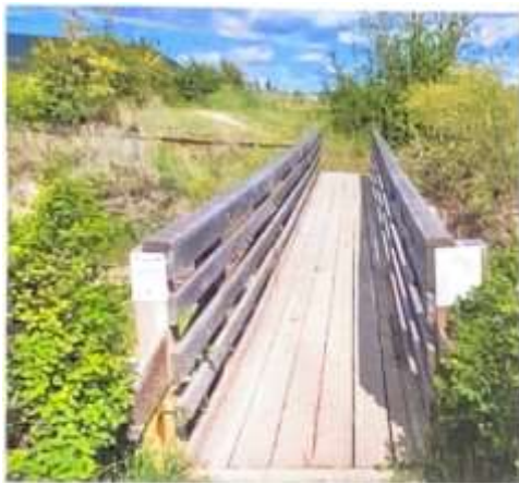
Present Otter Point Bridge
